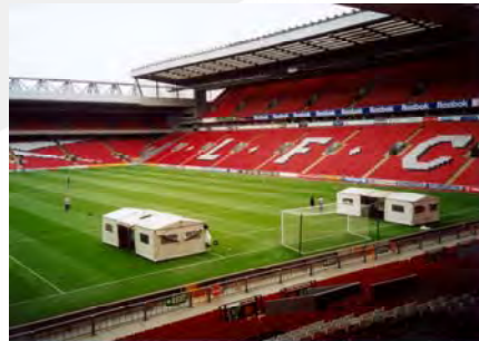
Installation Desso GrassMaster in Anfield Stadium, Liverpool FC
