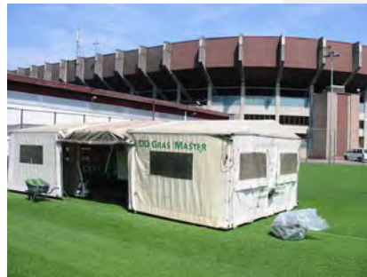
Installation of the Desso GrassMaster on the main training pitch of Sporting Anderlecht.
